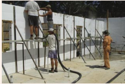
To wall construction
